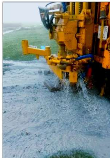
Figure 9. Image of drilling rig at site S-1.
