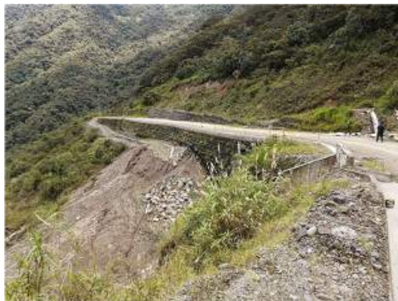
Figure 2. A view of the middle part of the landslide area where the road was affected (cut) and reconstructed, applying observed earth-walls. In this location, the movement is prone to continue at a low displacement tax. The high slope on the landscape can be observed.
